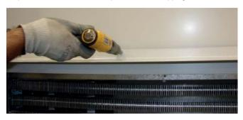
Step 3: insert the hose through the drill made for the connection to the indoor electric panel of the unit.
